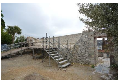
Reconstruction work nearing completion
