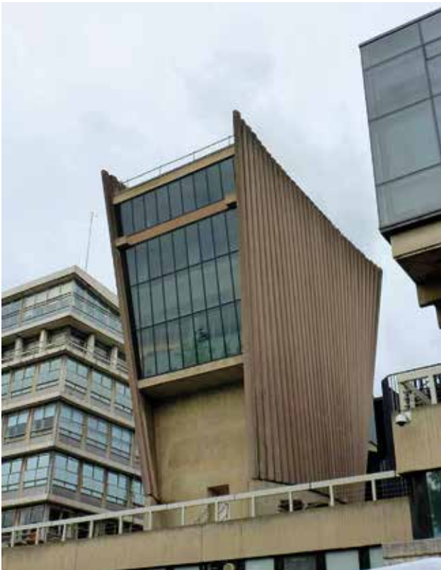
Fig 8 Tower of the Denys Wilkinson Building, University of Oxford
