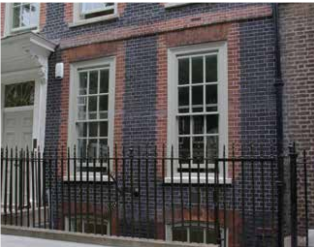
Fig 6 Detail of the restored front façade and railings, 2008
