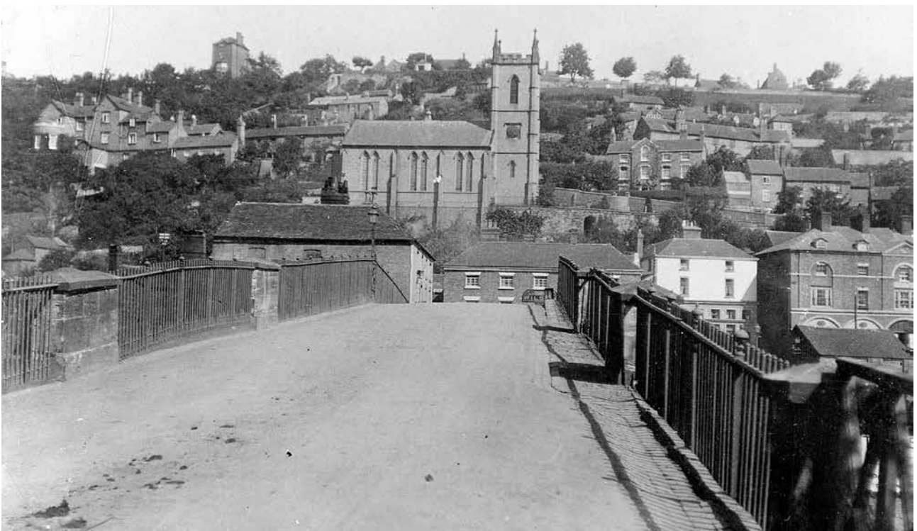
Fig 7 The roadway c1920 without footpath
