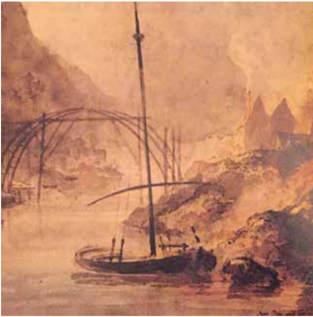
Fig 3 The Iron Bridge during construction (Elias Martin, 1779)
