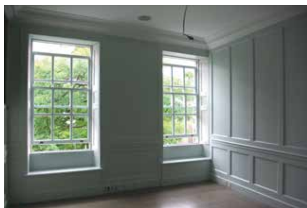
Fig 10 Repaired internal joinery, 2008
