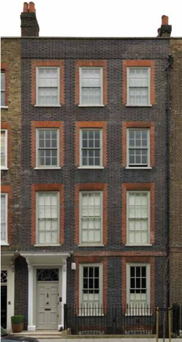
Fig 4 The front façade in 2013, five years after it was restored
