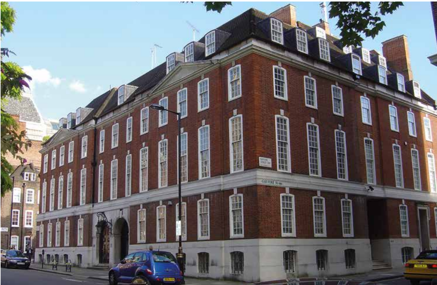
Fig 6 North House and Gayfere House, Gayfere Street, London
