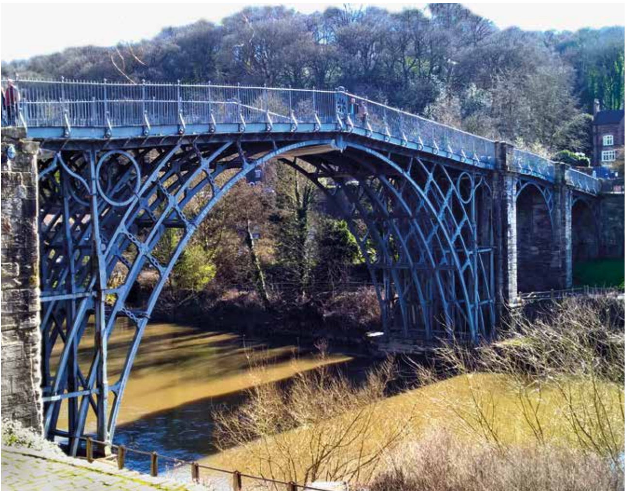
Fig 1 The Iron Bridge, Shropshire, upstream, west elevation
