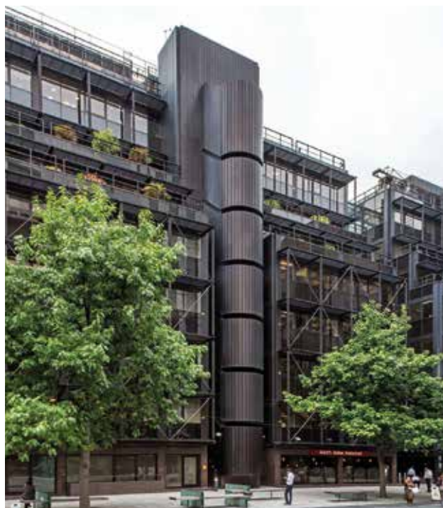
Fig 7 No 1 Finsbury Avenue, City of London, 1982-84
