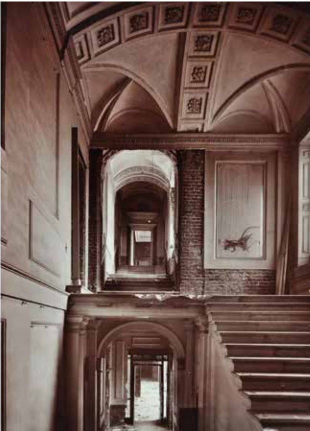
Fig 12 Harcourt House interior during demolition, 1906
