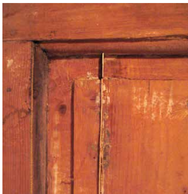
Fig 9 Detail of existing panelling under repair, 2008
