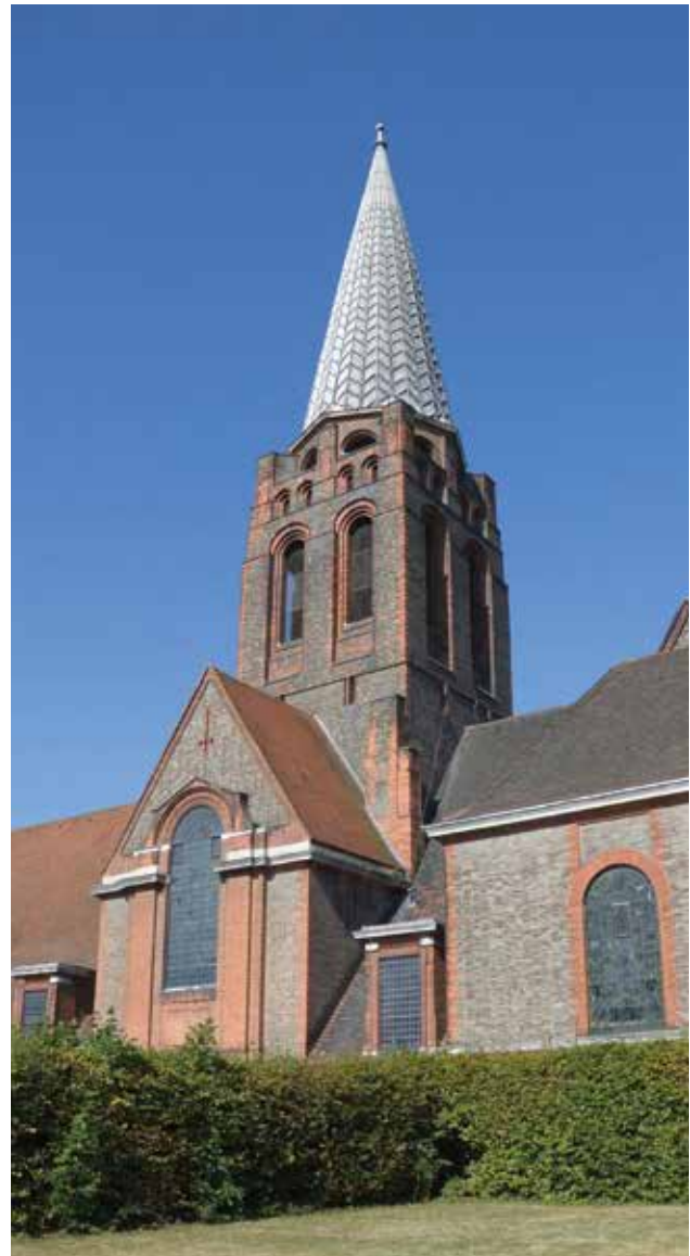
Fig 1 St Jude’s viewed from the south east
