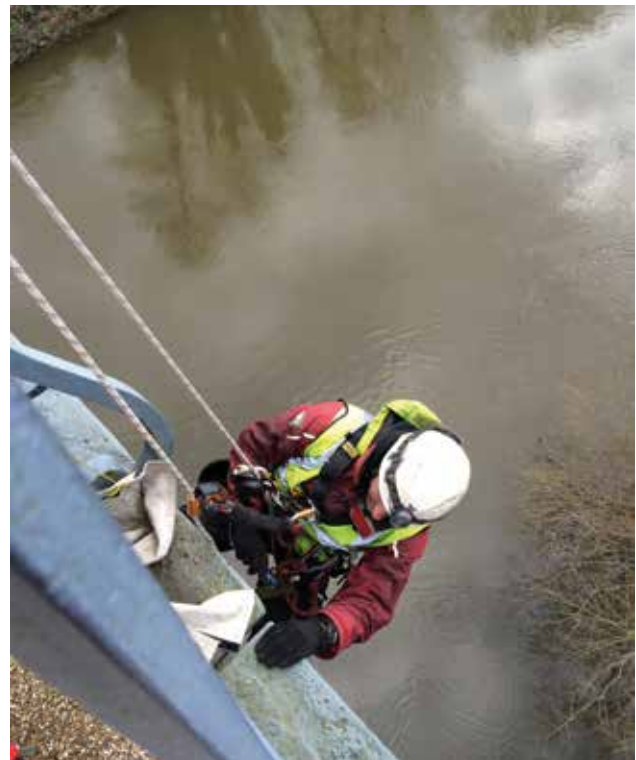
Fig 11 Roped access inspection being undertaken by Vertical Technology Ltd
