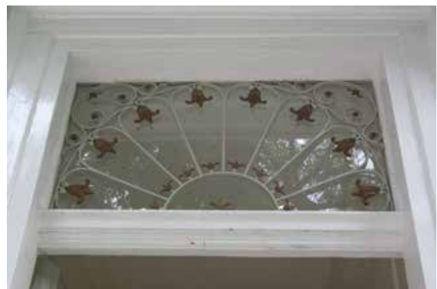
Fig 5 Restored fanlight over the front door, 2008
