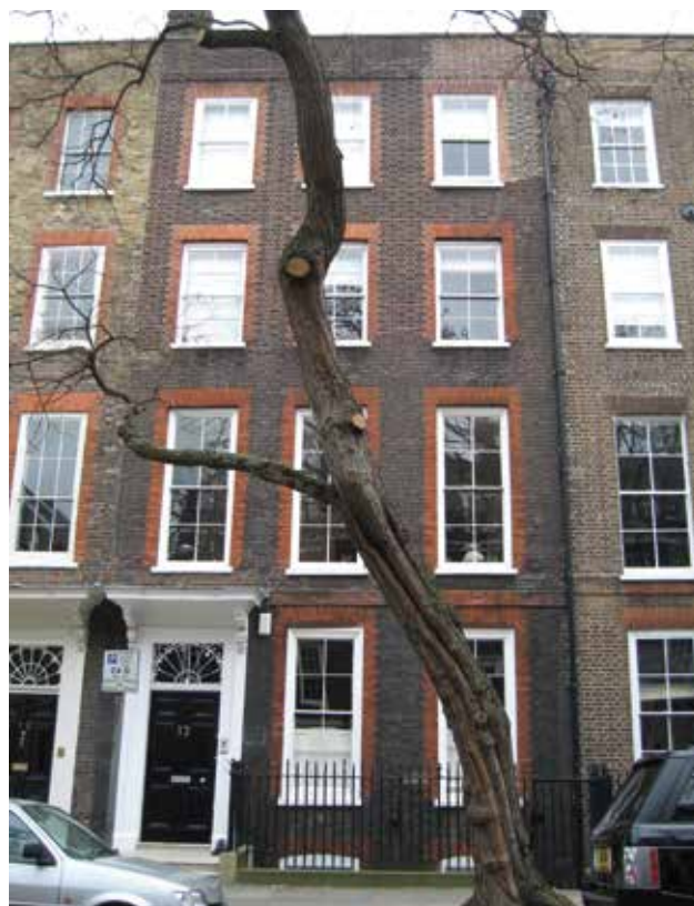
Fig 1 The front façade in 2008 before work began
