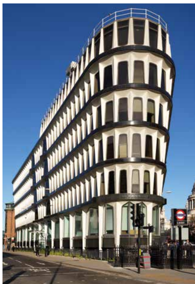
Fig 3 Credit Lyonnais, Cannon Street, City of London, 1974–77
