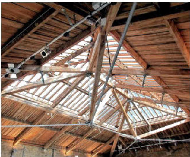
Fig 8 The roof of 34b York Way, now the Hub
