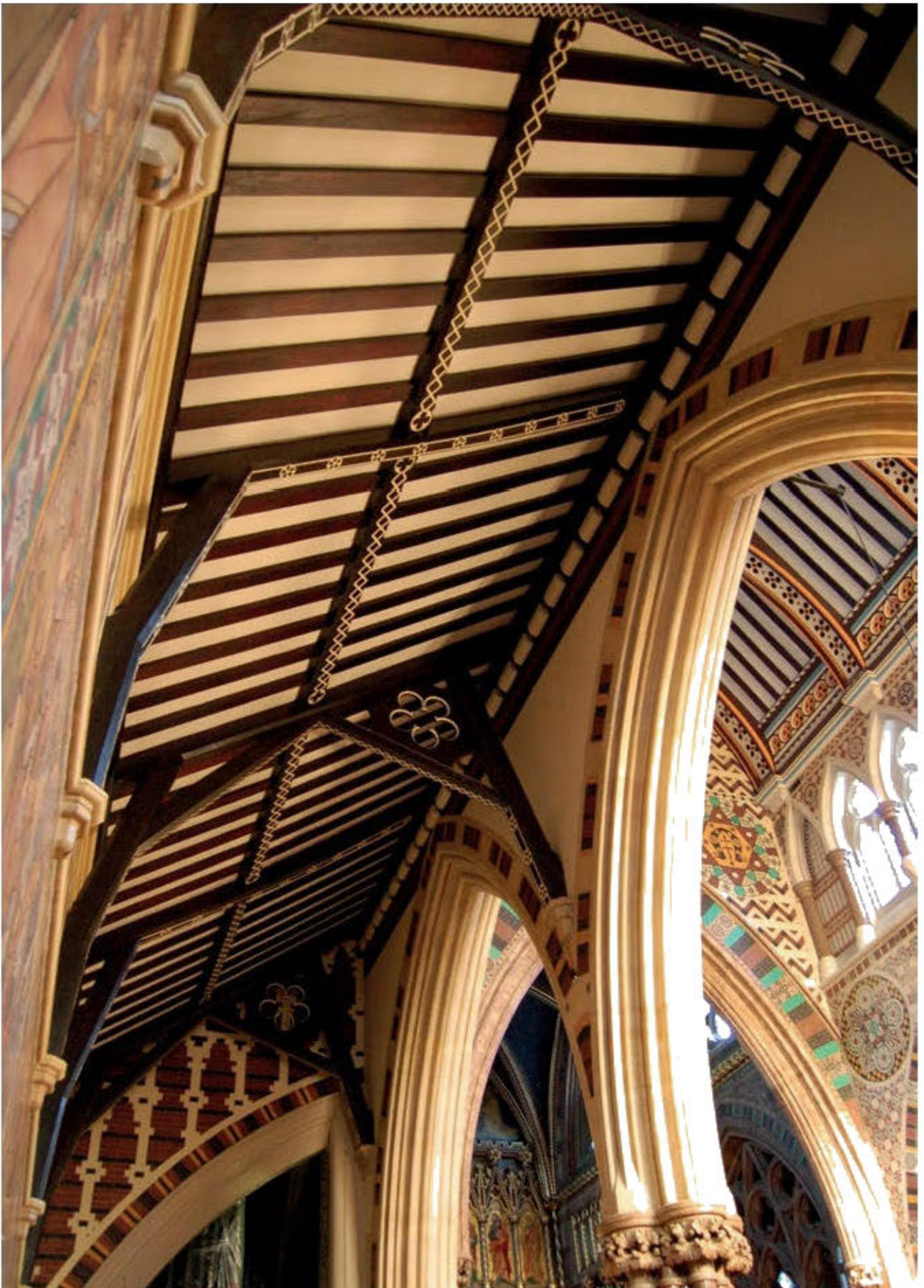
Fig 12 All Saints, restored aisle roof
