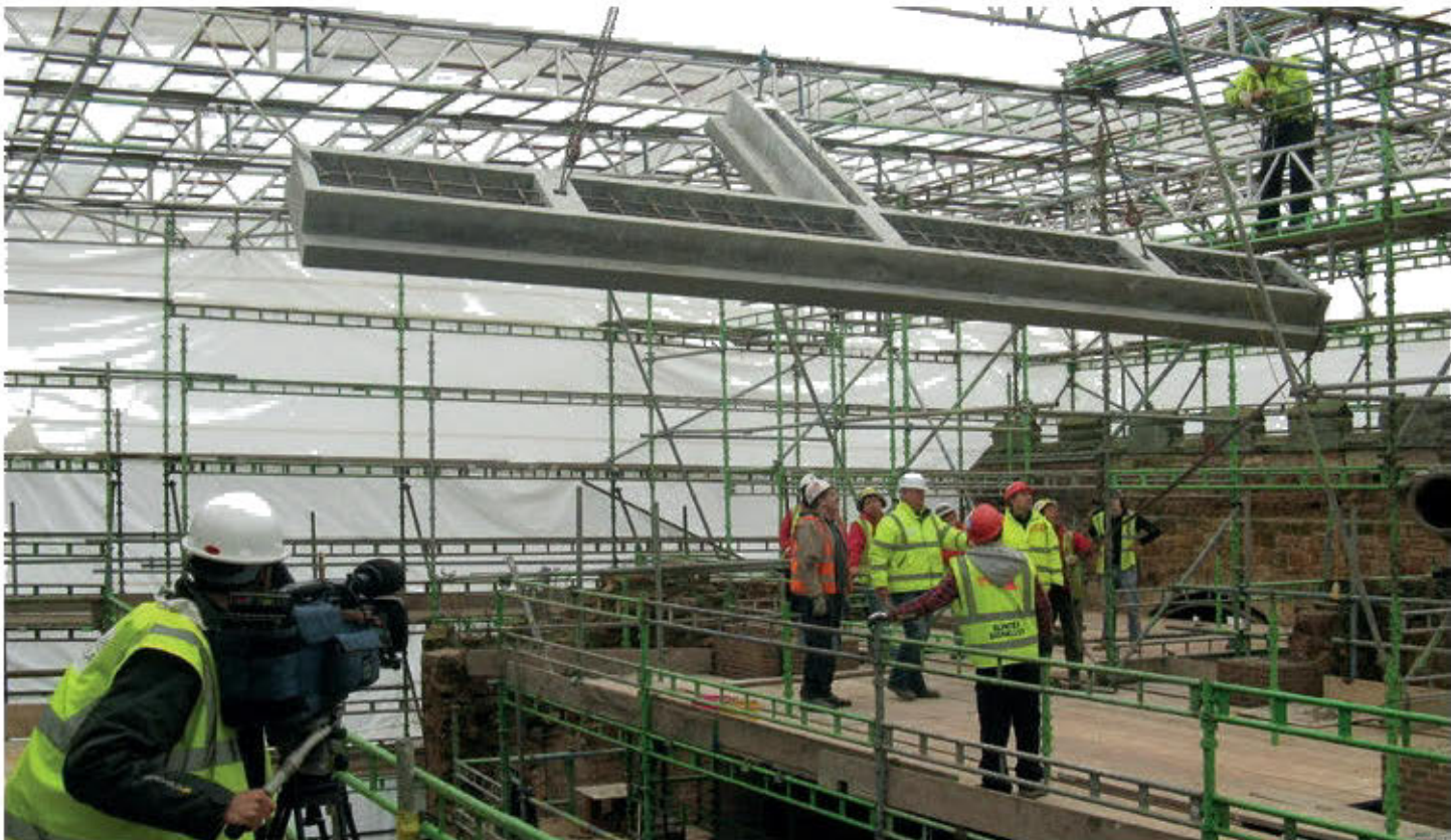
Fig 10 Installing the 'T' lintel
