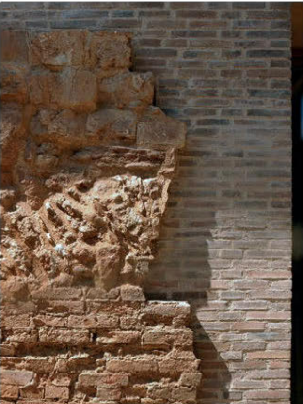
Fig 8 Junction of medieval and new brickwork
