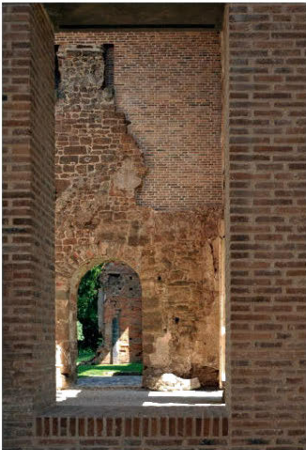
Fig 3 The south courtyard, 17th century construction
