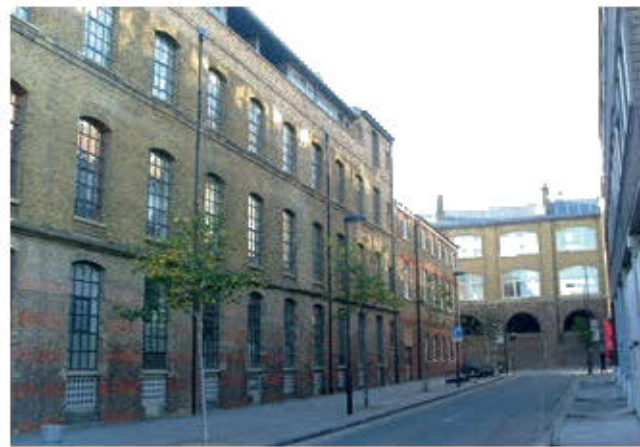
Fig 7 Former St Pancras Ironworks, after restoration and conversion
