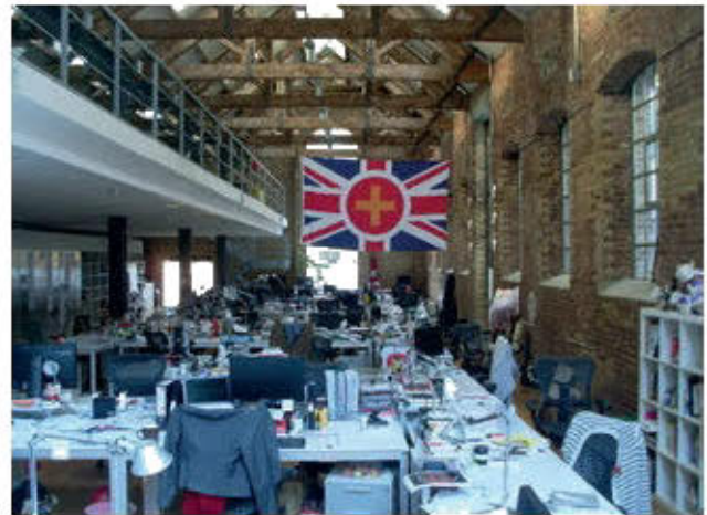
Fig 5 Interior of former Pontifex Copper and Brass Works
