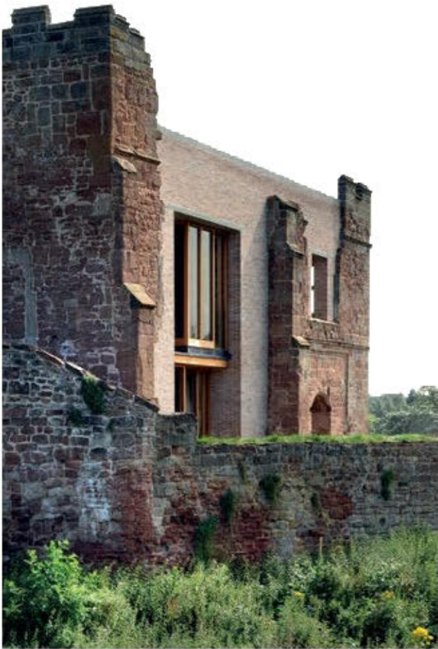
Fig 14 The castle from the southwest, showing stepped windows
