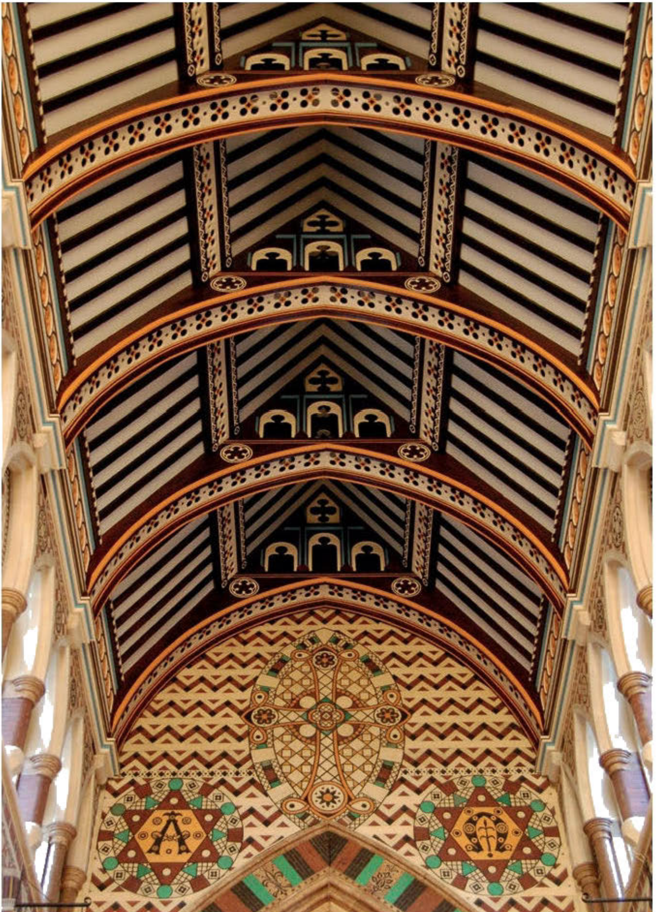
Fig 11 All Saints, the nave roof and chancel arch restored
