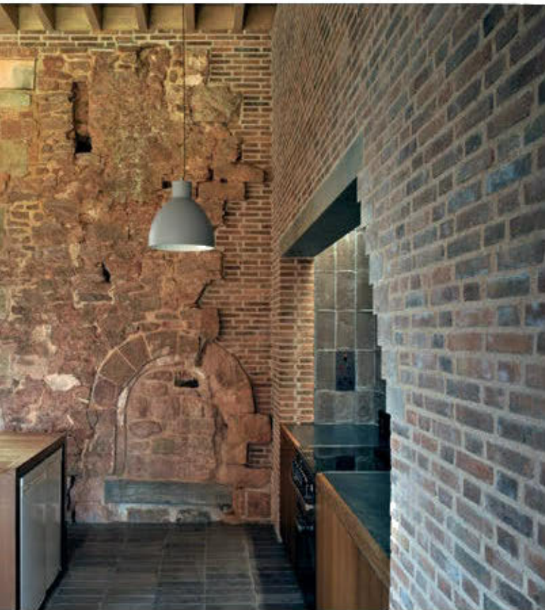
Fig 11 Stepped embrasure to the kitchen niche
