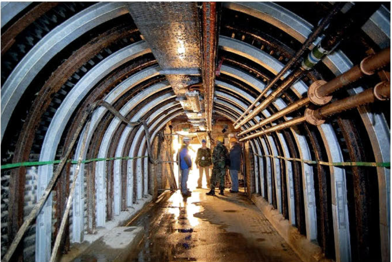
Fig 11 Mount Wise underground extension, Plymouth
