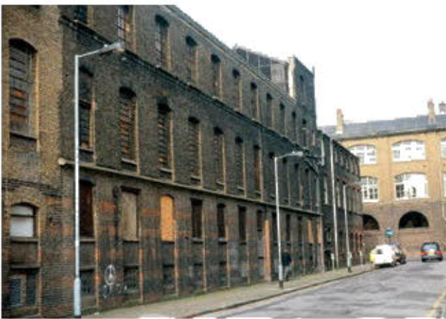
Fig 6 Former St Pancras Ironworks, vacant in 1999
