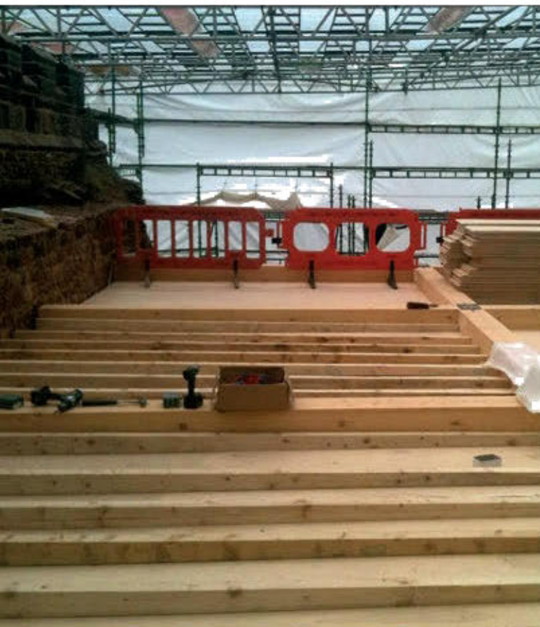
Fig 12 The roof in progress, showing upstand construction
