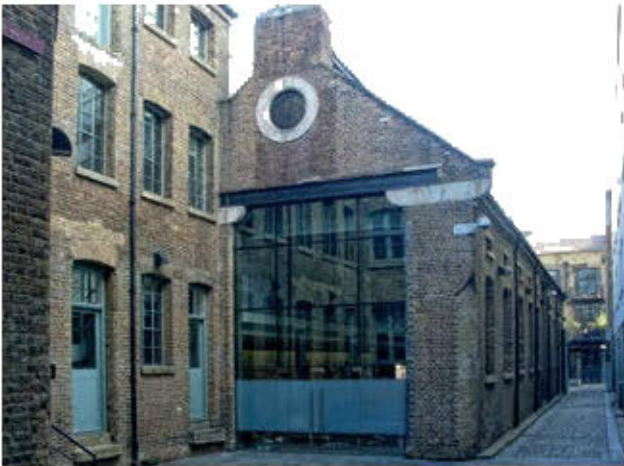
Fig 4 Former Pontifex Copper and Brass Works, converted to offices
