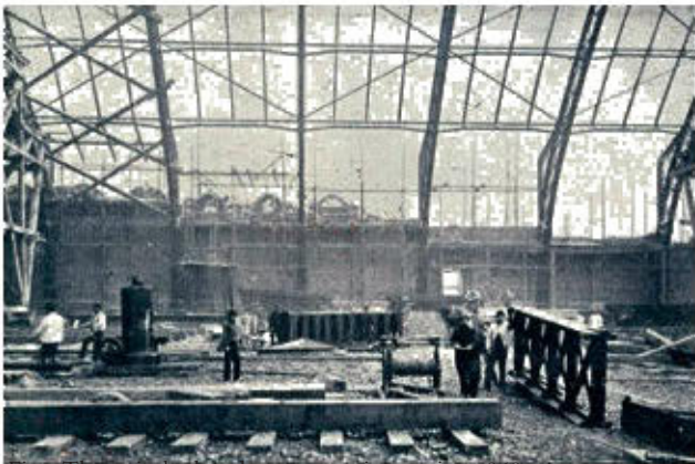
Fig 3 The trainshed under construction, spring 1868
