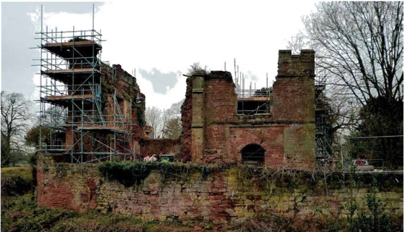
Fig 1 Astley Castle from the south in 2008, with stabilising work beginning
