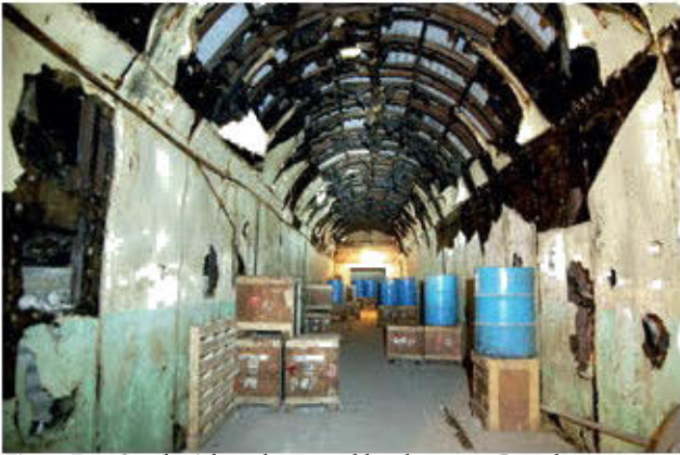
Fig 13 Fort Southwick underground headquarters, Portsdown
