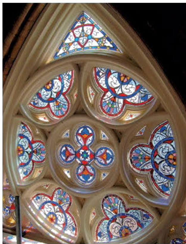
Fig 14 All Saints, restored clerestory window
