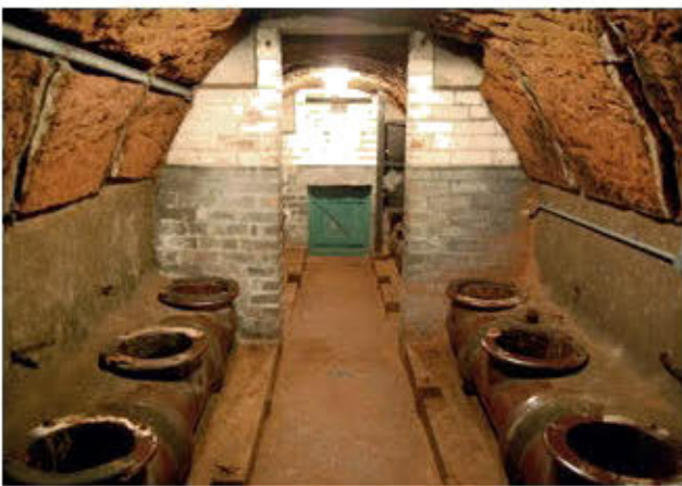
Fig 17 Toilets in Chestergate shelter, Stockport
