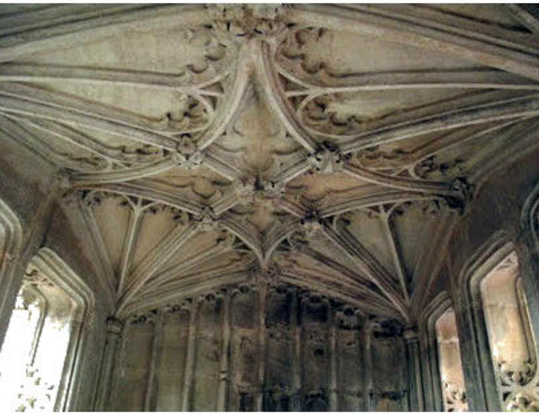
Fig 6 Underside of the vault after repair
