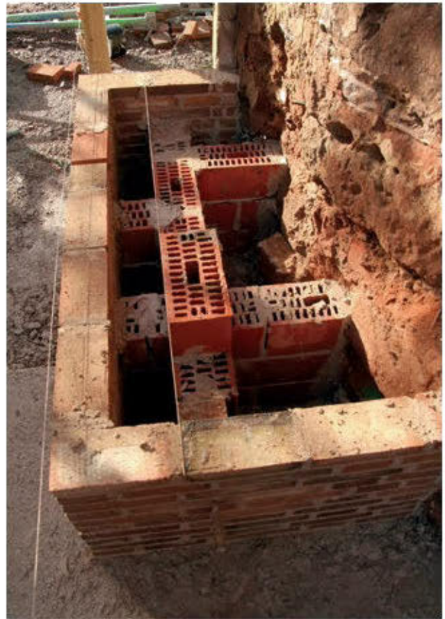
Fig 9 New brickwork and clay block diaphragms under construction
