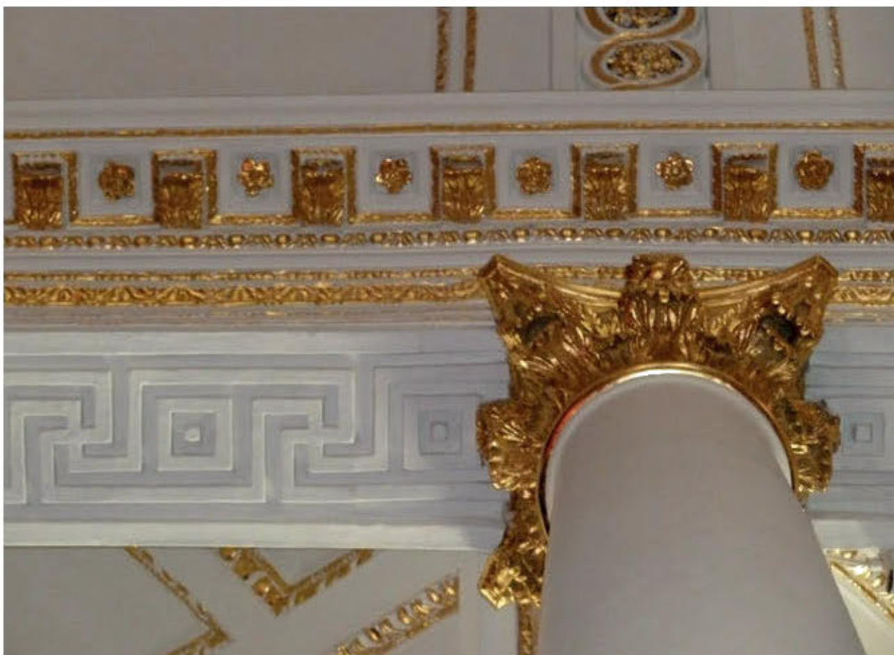
Fig 8 St George, re-gilding detail
