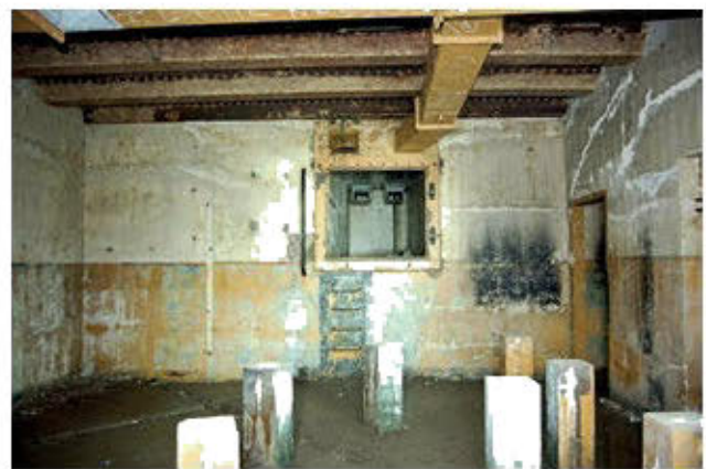
Fig 8 South Foreland plotting room, Dover
