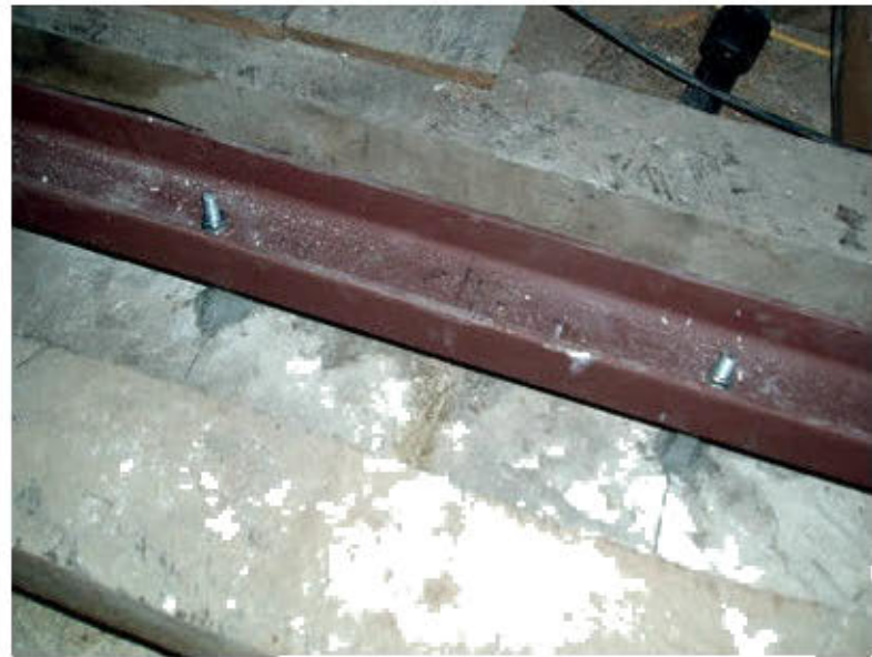
Fig 7 Steel beam within the floor structure
