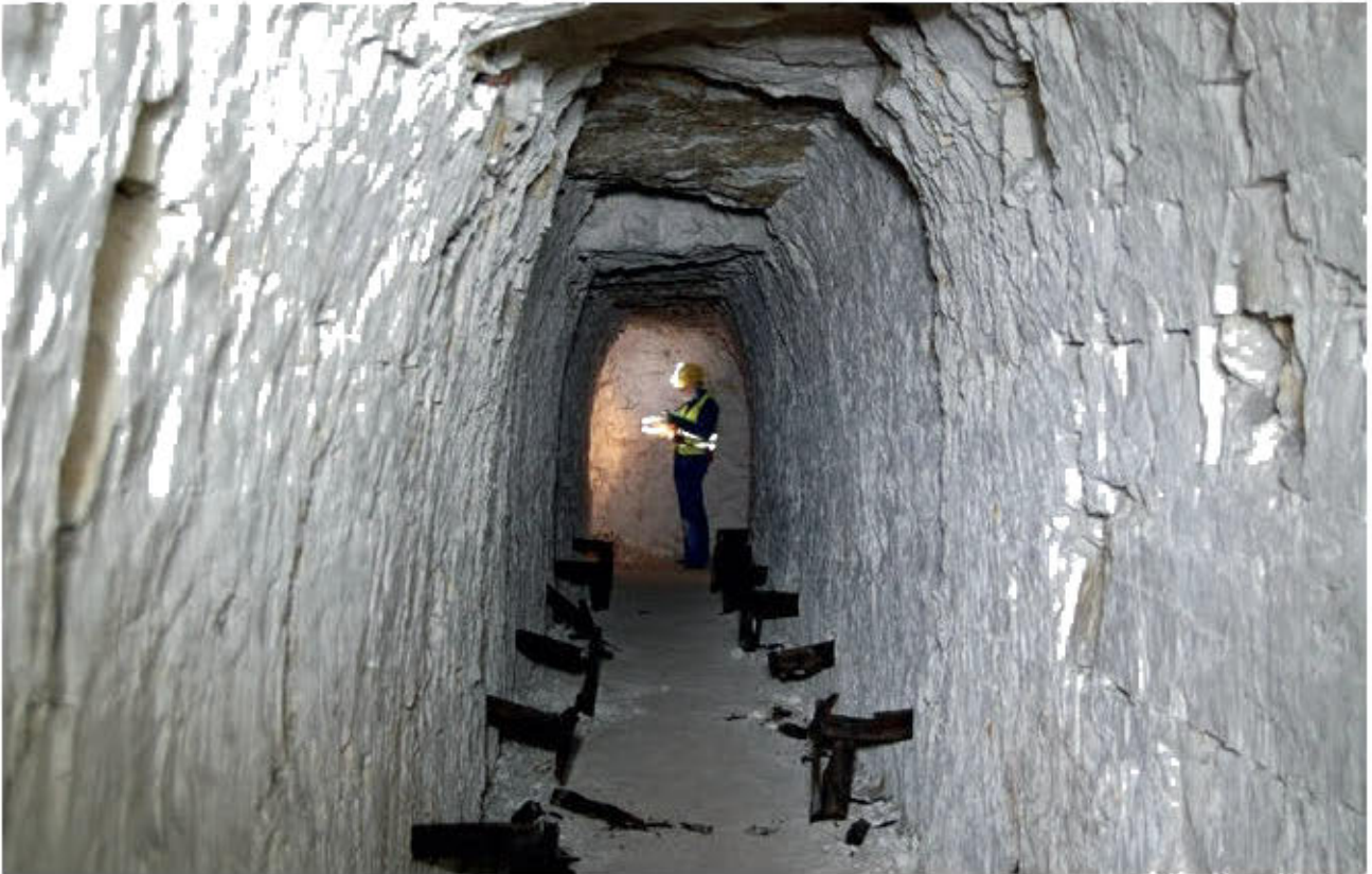
Fig 10 Ellington School shelter, Ramsgate
