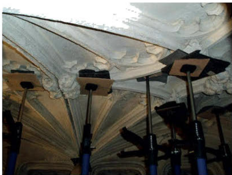
Fig 5 Propping and gently pushing the vault panels into place
