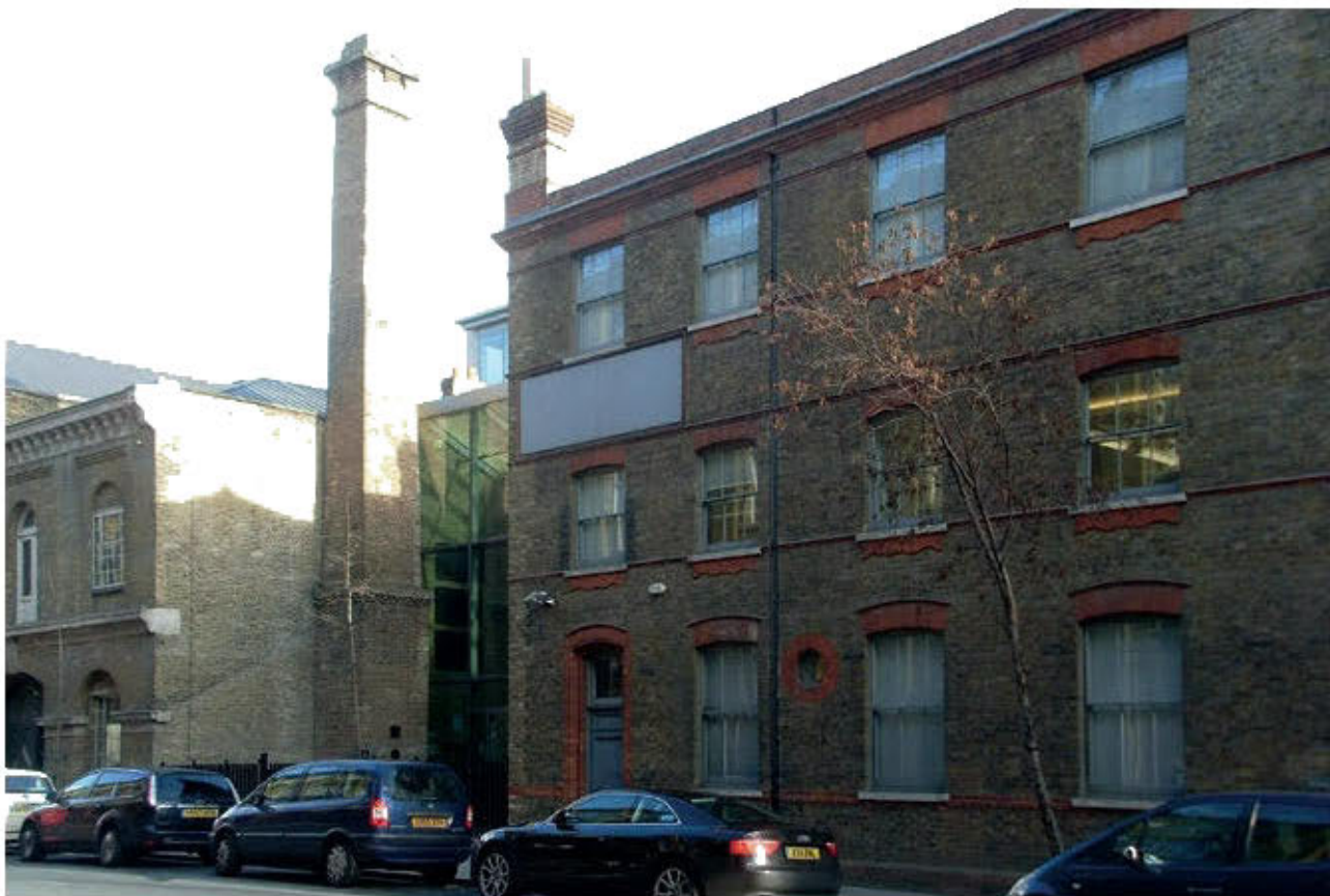
Fig 3 Jahn Building with frontage gap for new office entrance
