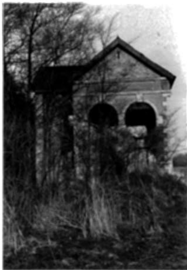
Figure 4 Stamford Grandstand from the west, March 1966. (RCHME)
