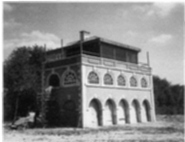
Figure 19 The render has been limewashed based on an analysis of the original ingredients, which included coppers; the newly glazed windows follow a traditional Stamford pattern; the chimney echoes a design of 1769. (Author)
