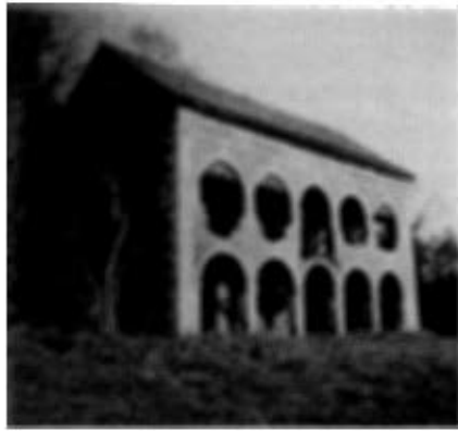
Figure 9 Stamford Grandstand, 1953, showing central arcade of upper storey lowered to form access to balcony of 1818–20. (Stewart Rodgers)
