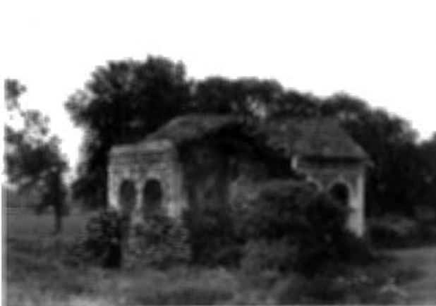
Figure 5 Stamford Grandstand from the south-west, June 1981. (RCHME)
