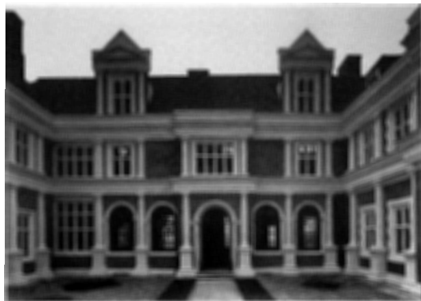
Figure 8 The South Courtyard Elevation after restoration, with new Corinthian dormers and dais window.
