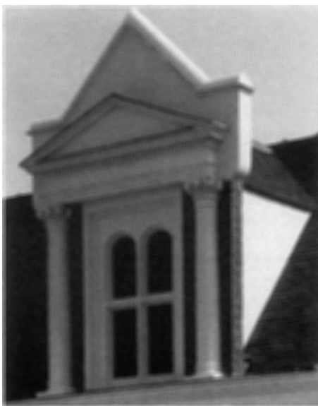
Figure 18 The Corinthian dormer with completed plaster finish.
