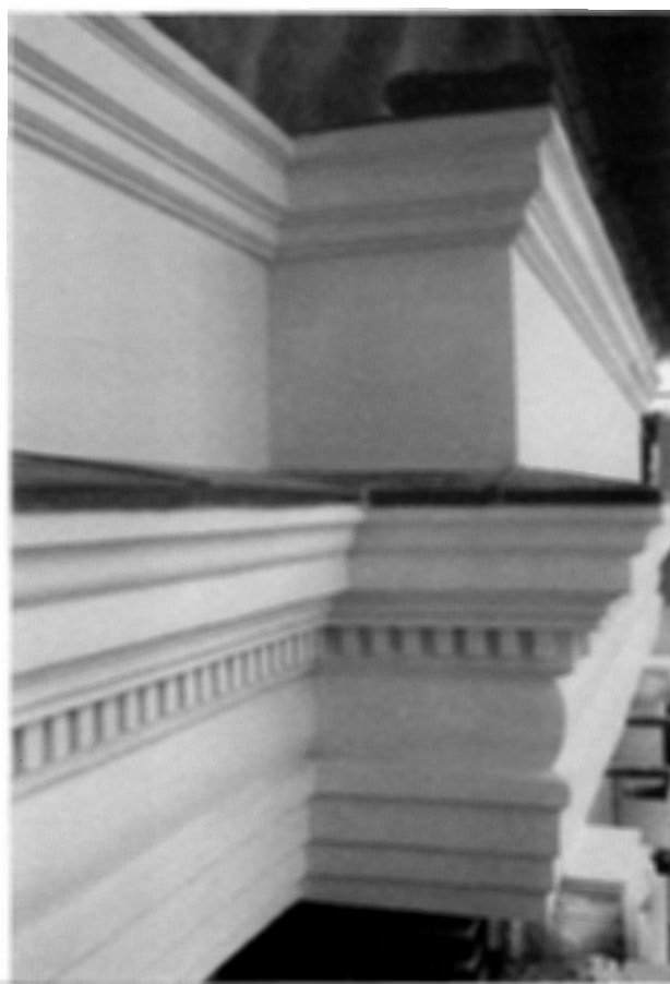
Figure 14 The fine lime plaster finish, without limewash, to the Ionic entablature.
