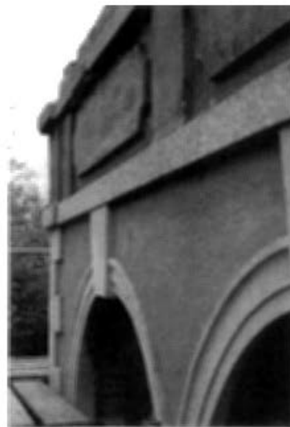
Figure 11 Close-up of ashlar dressings in north arch and render on parapet of west face of main block. (Donald Mackreth)
