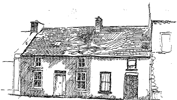
Figure 17 Houses in Killough, Co Down (1980). Ulster towns were once full of modest single- and two-storey 19th-century houses like this, with their first floor windows squeezed under the eaves. Most have been cleared in the last thirty years as part of housing improvement schemes.
