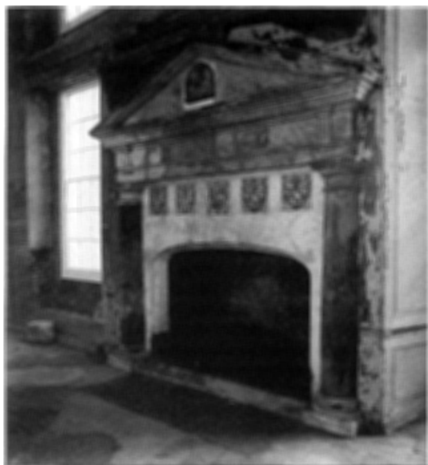
Figure 28 The Great Hall chimneypiece during conservation. The original grey plaster has been repaired on the columns with a matching mix, which is still drying out.
