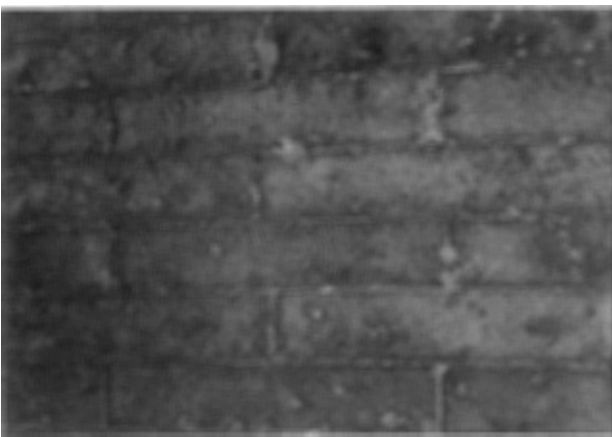
Figure 1 Herringbone tool marks from post-fired finishing on bricks at Santa Maria Della Scala, Siena, Italy. Note the fineness of the joints, made possible by the 'ashlaring' of the bricks to sharp arrises.
