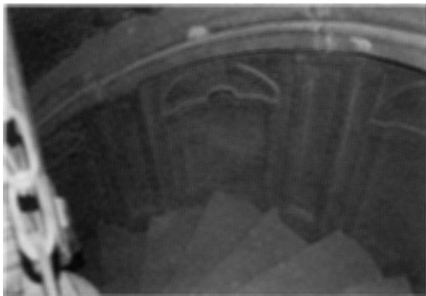
Figure 10 A section of the seventeenth-century gauged brickwork masterpieces in De Waag, Amsterdam, that follow the spiral staircase to the top of the entrance tower in De Waag, Amsterdam.
