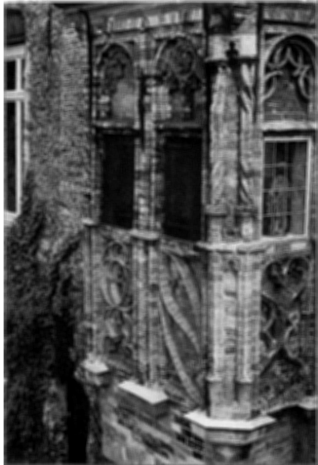
Figure 5 Wonderful early Flemish decorative gauged brickwork at Tribune Hereman van Outvelde, Brugge.
