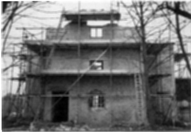
Figure 16 Stonework at rear of stand under repair, Winter 1995; timber lintel of door opening and case windows are of 1766. (Author)
