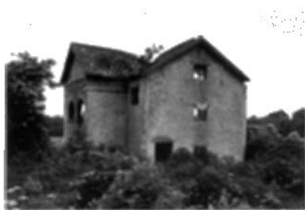
Figure 6 Stamford Grandstand from the north-east, June 1981. (RCHME)
