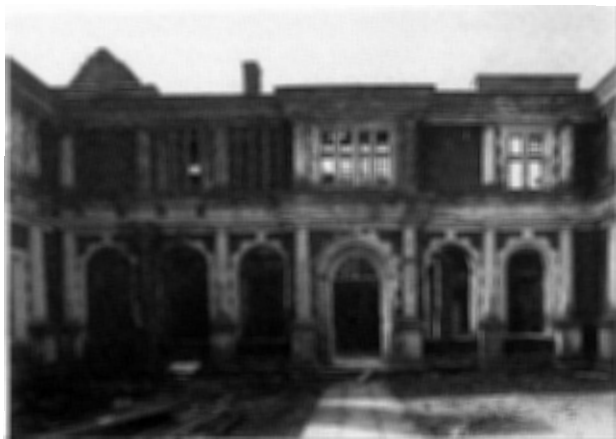
Figure 7 The South Courtyard Elevation before restoration.
