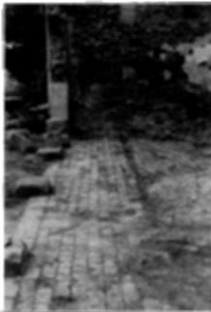
Figure 13 Brick paving revealed in view looking west of padstones of south arcade; slot in brick floor may have held partition for counter; stones set between arches possibly reduced by wear. (Donald Mackreth)
