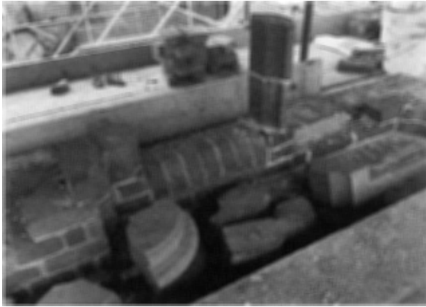
Figure 17 Setting out the base of the Corinthian dormer.
