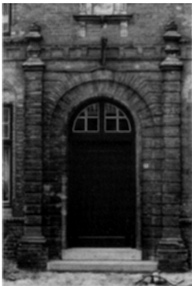
Figure 6 Fine gauged brickwork doorway, built of stone-like buff-coloured coastal bricks, at 71 Gasthuisstraat, Poperinge.
